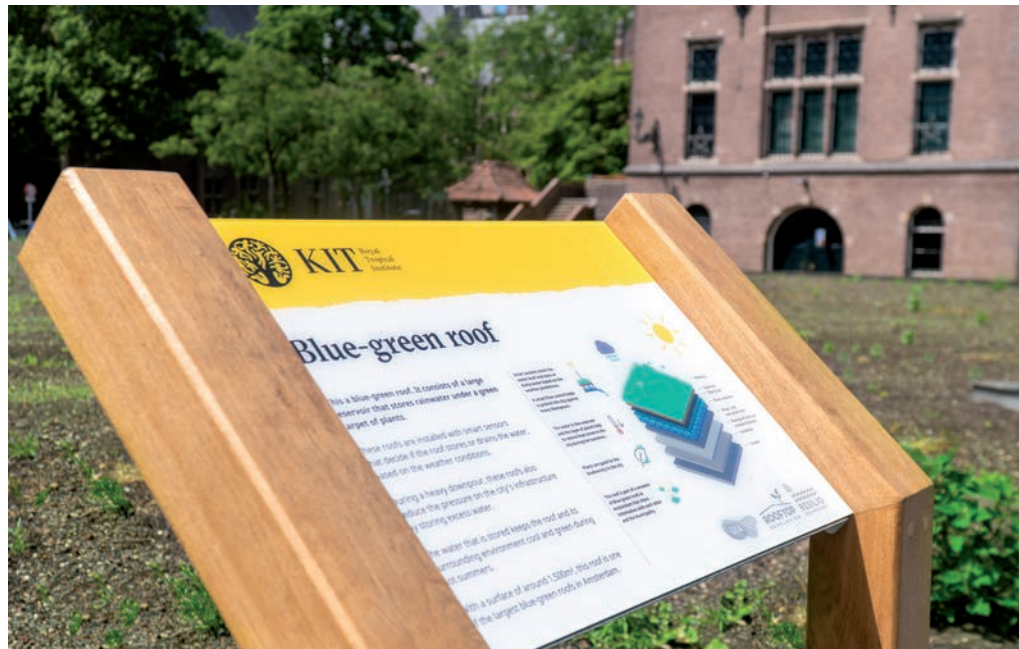
Above the depot of the Tropenmuseum, we installed a blue-green roof last summer. Blue-green roofs store or dump water based on weather predictions, helping manage use during periods of droughts or heavy rainfalls.
